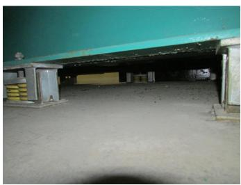
**HS1 View 3** - concrete floor condition underneath emergency generators
