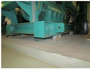
**HS1 View 1** - concrete floor condition underneath emergency generators
